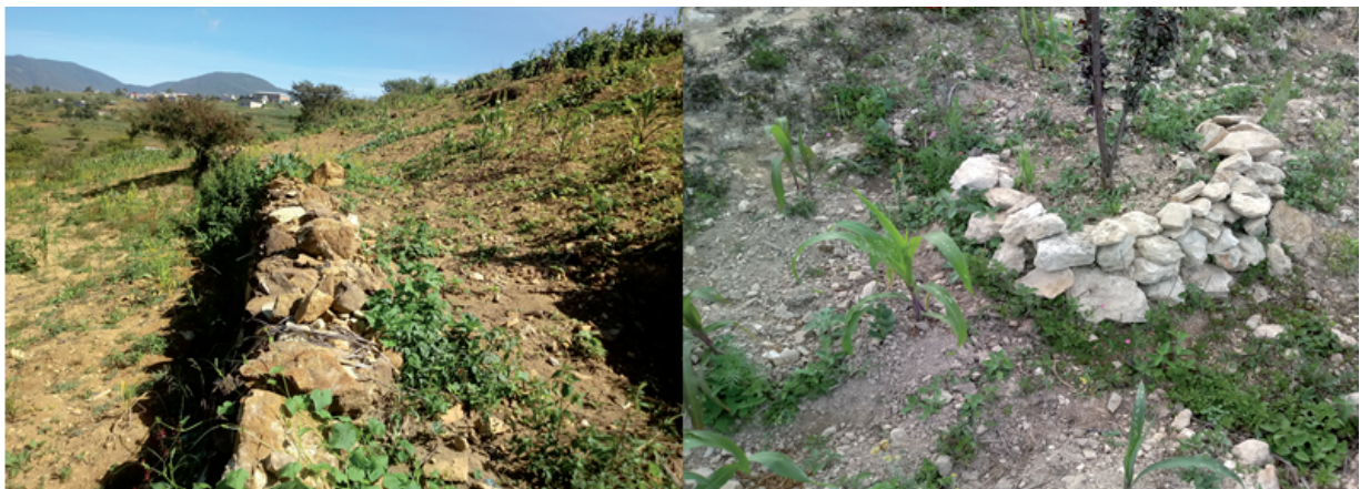
Figure 1. Retention walls in Yareni (left) and individual terraces in Abejones (right).
